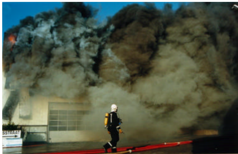
Empty Building = No internal Fire load
